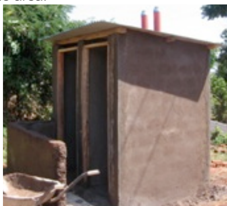
A freshly plastered latrine, ready for painting.
