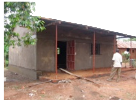
Our biggest project of the year, near completion.
