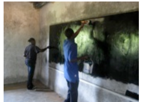
Local volunteers help paint the blackboards inside the new building.
