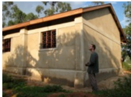
Kevin admires the new building we constructed to replace that sad structure at the top of the page. Something of an improvement, don't you think?
